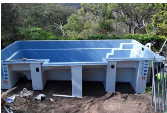
Start of installation
